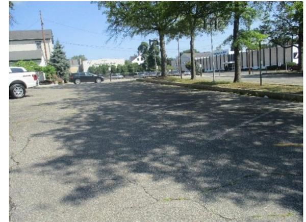
Parking spaces can be replaced with porous asphalt to capture and infiltrate stormwater runoff. A preliminary soil assessment suggests that the soils have suitable drainage characteristics for green infrastructure.
