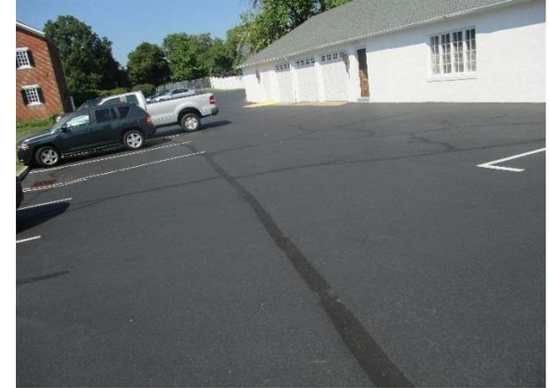
Parking spaces can be replaced with pervious pavement to infiltrate parking lot runoff. A preliminary soil assessment suggests that the soils have suitable drainage characteristics for green infrastructure.
