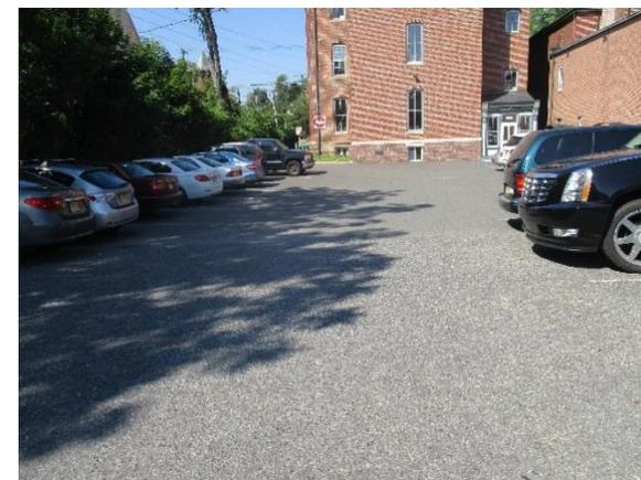
Parking spots by the north building can be replaced with porous asphalt to infiltrate stormwater. A preliminary soil assessment suggests that the soils have suitable drainage characteristics for green infrastructure.
